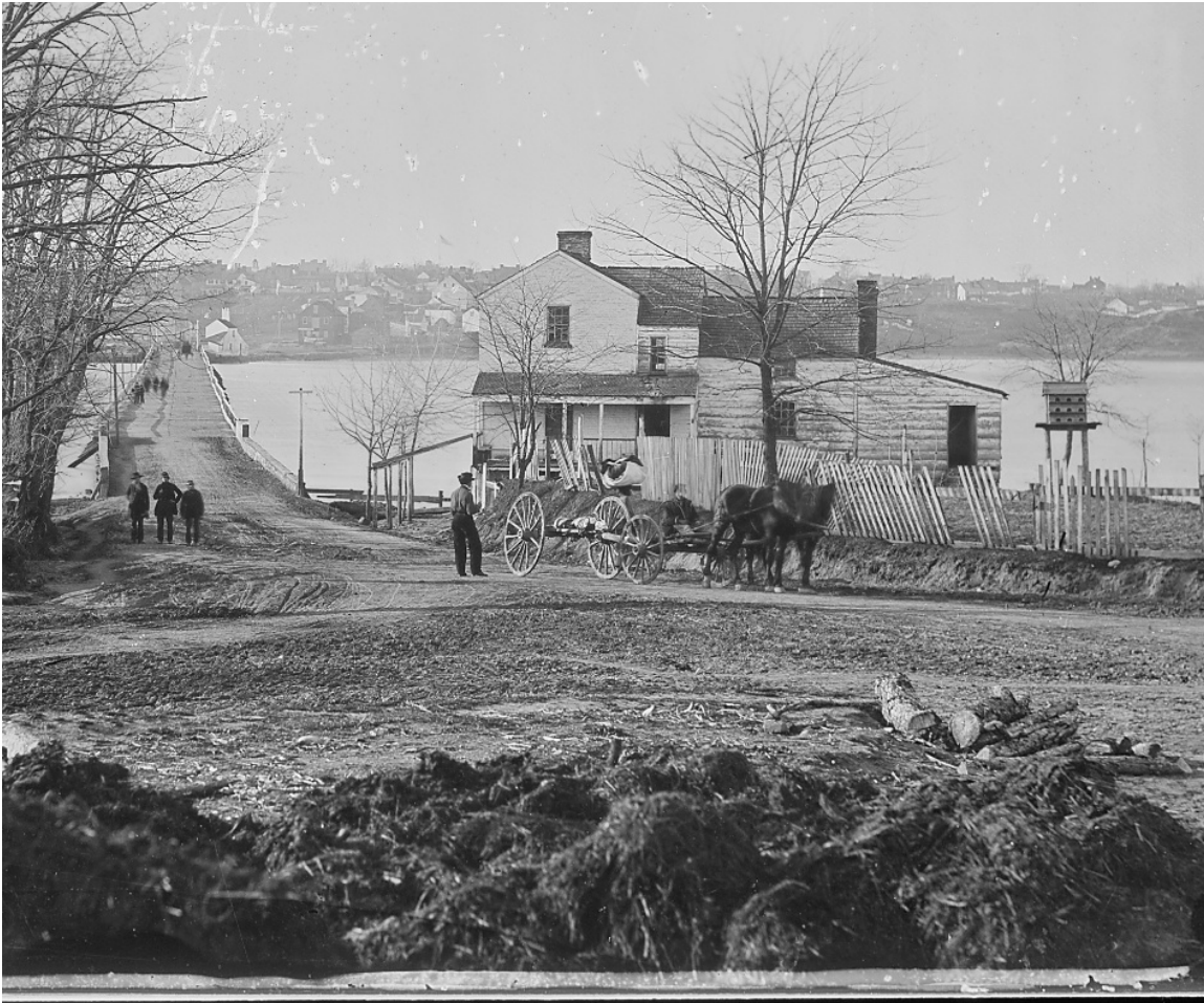
Matthew Brady Photograph of Bridge Over the East Branch, Wasington, DC, 1862. Note the purple martin box in the yard to the right of the house.
