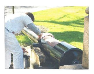
In 2001, volunteers from the International Painters Union removed the cannons and completely restored them, removing corrosion and old paint (including dead birds and beer cans from the bores). The work had to be done by hand and took over 6 months. The results are outstanding – the surfaces are smooth and finished as original. Best of all, the markings are clear and legible.
